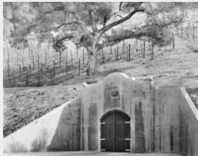
THE NEWLY COMPLETED WINE CAVE 2003 PHOTO BY OLAF BECKMANN
